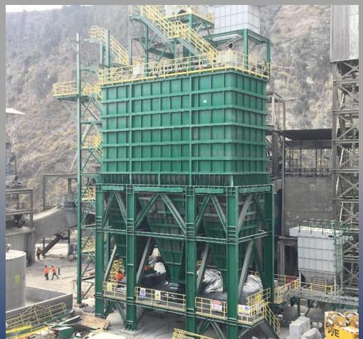
Customer: GEBR. PFEIFFER USA Remarks : Detailed design and fabrication of cement plant's steel structures. (400 tons)
