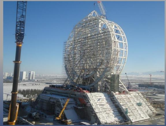
Customer: POLİMEKS Turkey Remarks : Design, fabrication and erection of 65 m diameter, 115 m height ferris wheel- 2.000 tons.
