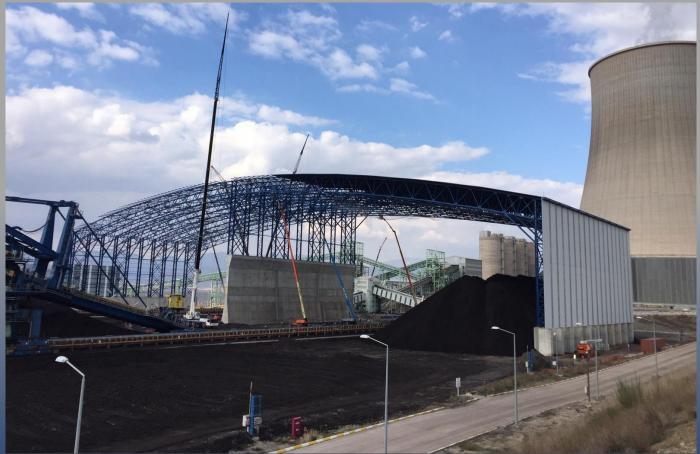
Customer: ENERJİSA Turkey Remarks : Detailed design, fabrication and erection of roof steel structure and including all roof and cladding, civil, structural works. (2.100 tons)
