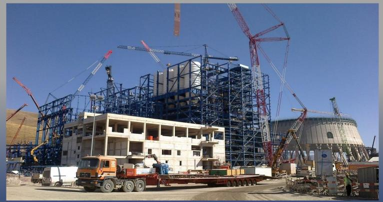
Customer: SK GROUP Korea Remarks : Fabrication of 7.650 tons steel structure of the steam turbine building. Date of completion: 2014
