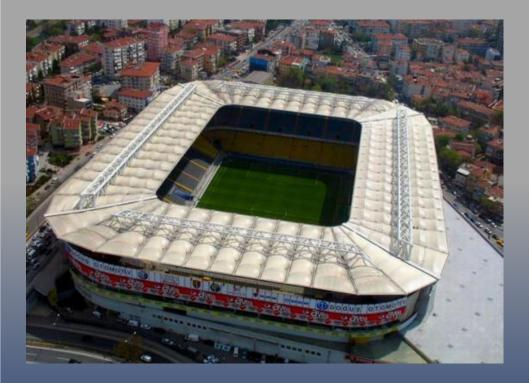
Customer: Fenerbahçe Sports Club Turkey Remarks : Design, fabrication and erection of roof structure 1700 tons.
