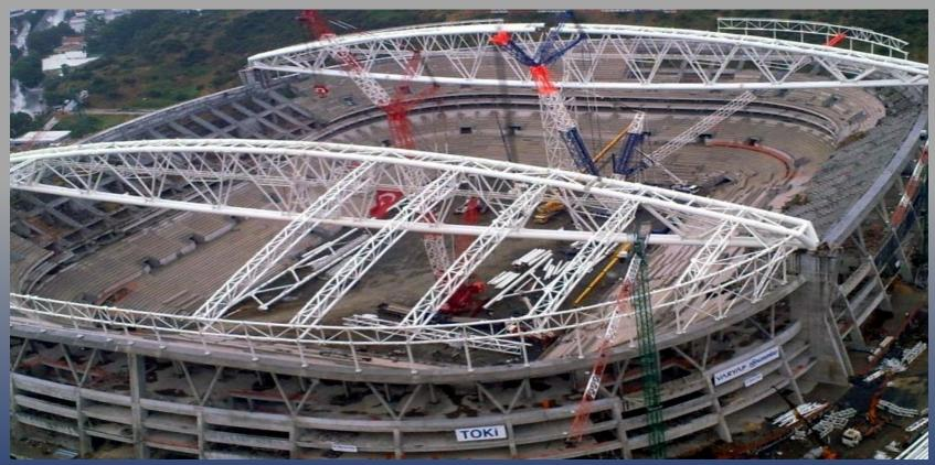
Customer: Varyap-Uzunlar JV Turkey Remarks : Design, fabrication and erection of roof steel structure of Seyrantepe Stadium. (6.000 tons) Date of completion: 2010
