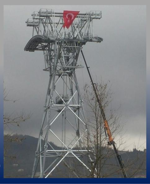
Customer: Leitner Italy Remarks : Fabrication and erection of structural steel ropeway towers in Trabzon -Turkey. (600 tons) Date of completion: 2017
