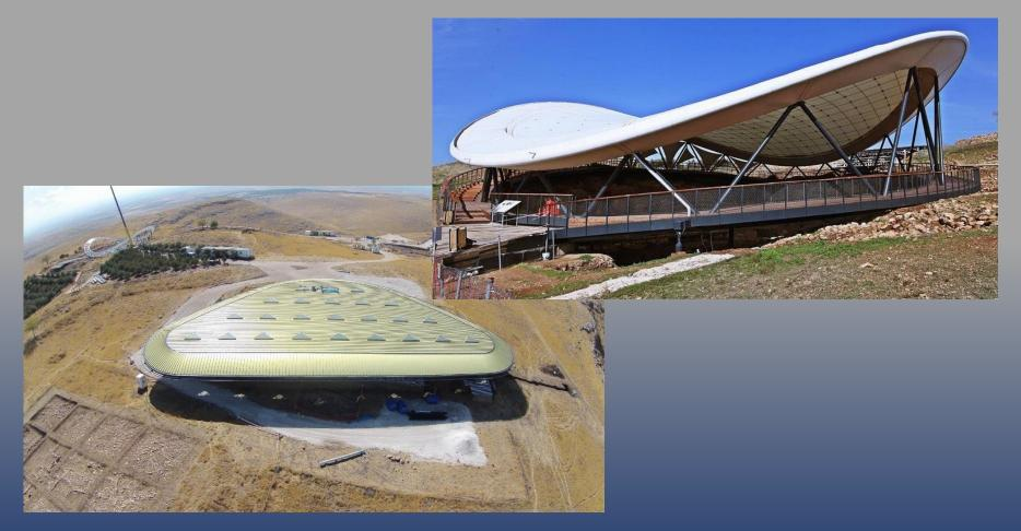
Customer: Trans-t Construction Turkey Remarks : Detailed design, fabrication and erection of roof structural steel in Şanlıurfa- Turkey. (500 tons)
