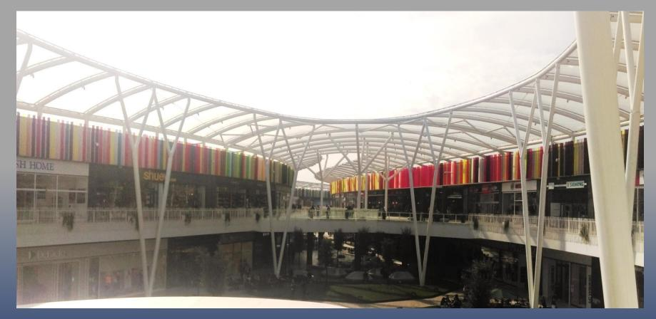
Customer: Vector Foiltec Germany Remarks : Fabrication and erection of İzmit shopping mall steel structure in İzmit. (650 tons) Date of completion: 2015
