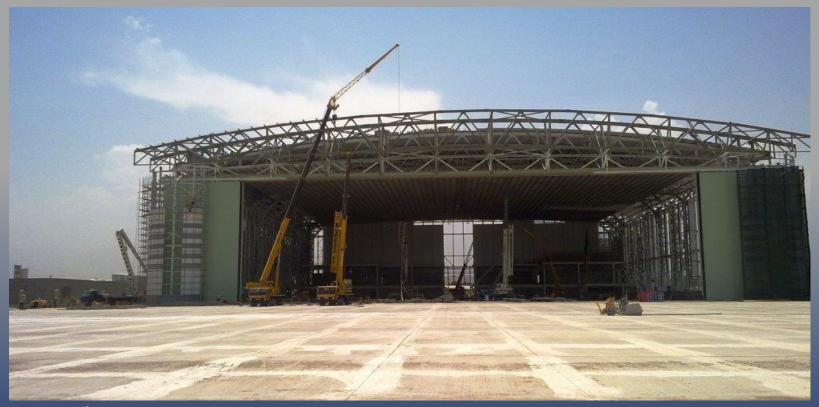
Customer: POLİMEKS Turkey Remarks : Design, fabrication and erection of 3600 tons steel structure
