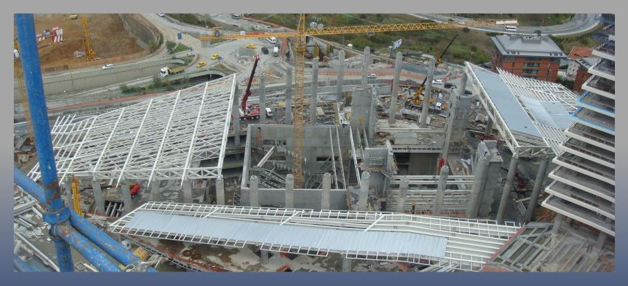
Customer: Aktürk Construction Turkey Remarks : Fabrication and erection of the steel theatre roof of the Zorlu Center (5.500 tons) Date of completion: 2012
