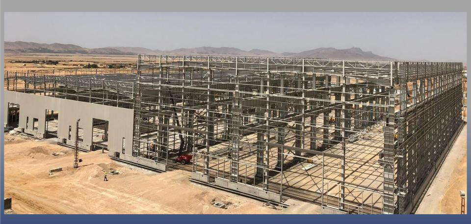
Customer: Renaissance Construction Turkey Remarks : Fabrication and erection of the structural steel of the Turbine Factory in Algeria. (5.500 tons) Date of comletion: 2018
