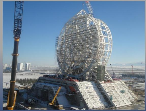
Customer: POLİMEKS Turkey Remarks : Design, fabrication and erection of 65 m diameter, 115 m height ferris wheel- 2.000 tons.
