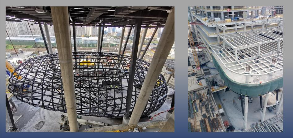
Customer: KALYON Turkey Remarks : Detailed design, fabrication and erection of the towers and auditorium steel structure works. (2.200 tons)
